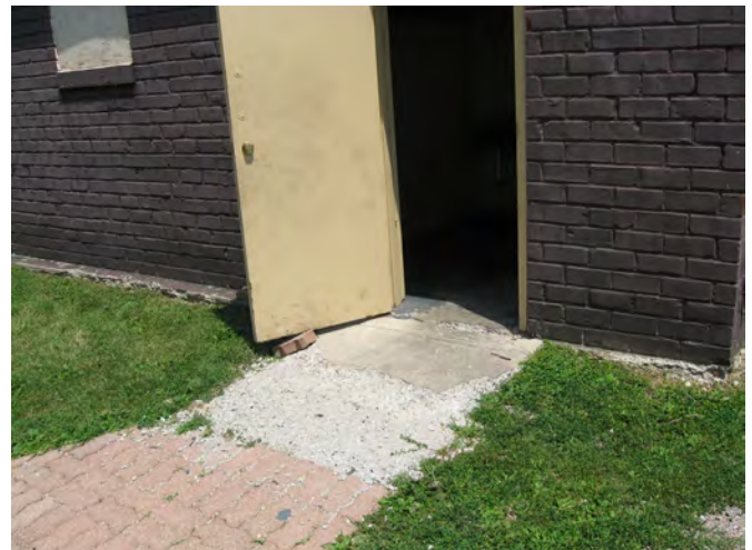
Concrete Pad at Men's Restroom Door
