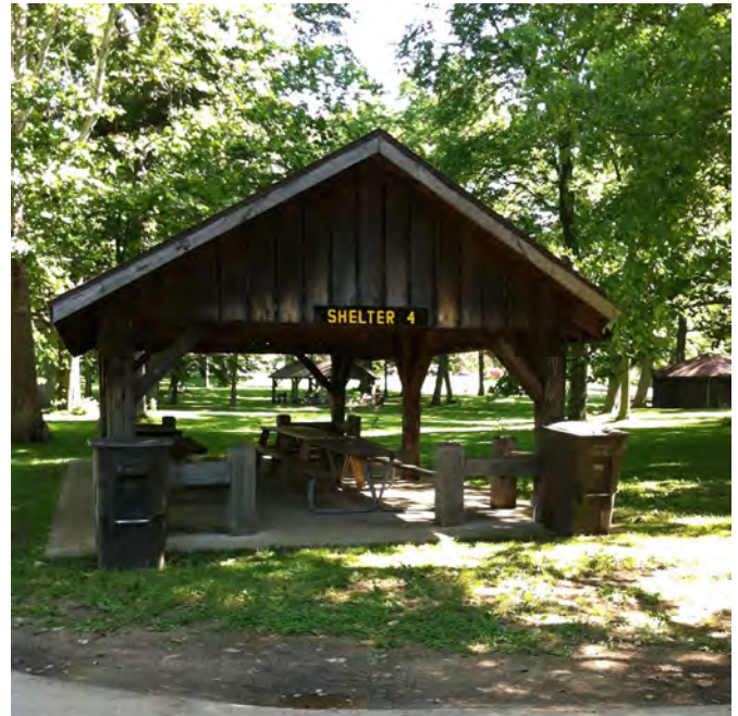
Shelter 4 with Shelter 3 and restrooms in background
