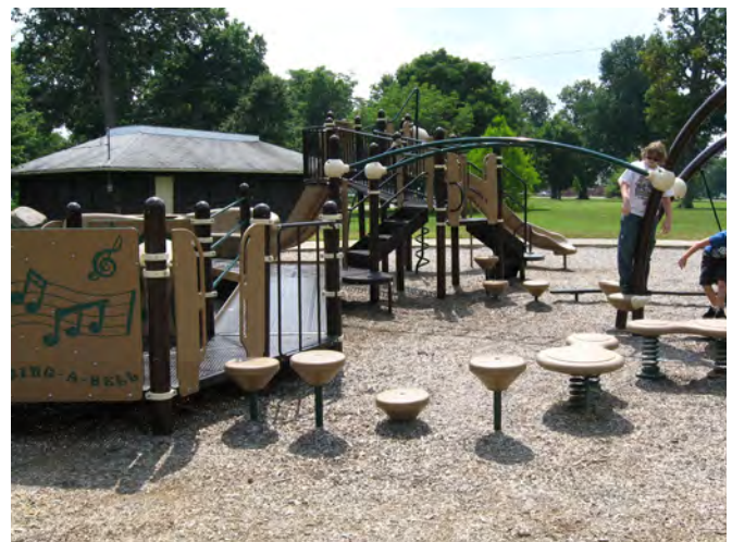
Ramped and ground level play components on composite play structure. Transfer steps to additional elevated play components can be seen on the far unit.
