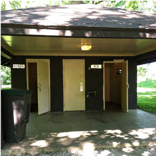
Restroom building with attached drinking fountain
